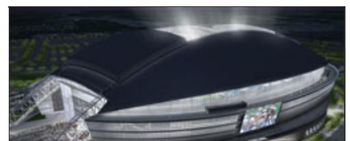
structural steel. At 661,000 sq ft, the stadium's domed roof will be the largest in the world. The retractable roof design includes two bi-parting mechanized roof panels, each measuring 63,000 sq ft. They will be opened and closed with a rack-and-pinion drive system.
