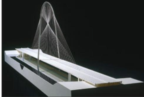
The signature cable-stayed bridge, which is the first vehicular bridge in the U.S. designed by renowned Spanish architect Santiago Calatrava, features a dramatic 395-ft-tall central parabolic steel arch. Cables fan out from the arch to support the deck of the 600-ft-long clear span. The official groundbreaking was in December 2005, and Williams Brothers, Houston, expects to complete the project by August 2009.
